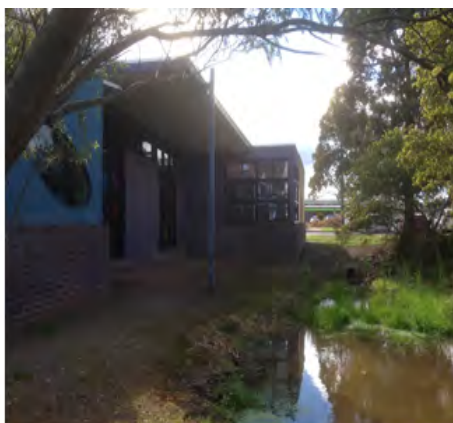
The art room at Boardwalk where a doorway will be built to lead onto a new deck. At this point there is a pond, formed in the swale.
